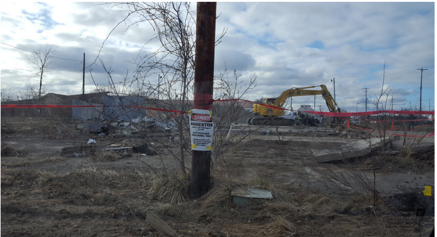
Genesee Charter Township - Demolition - $49,056
