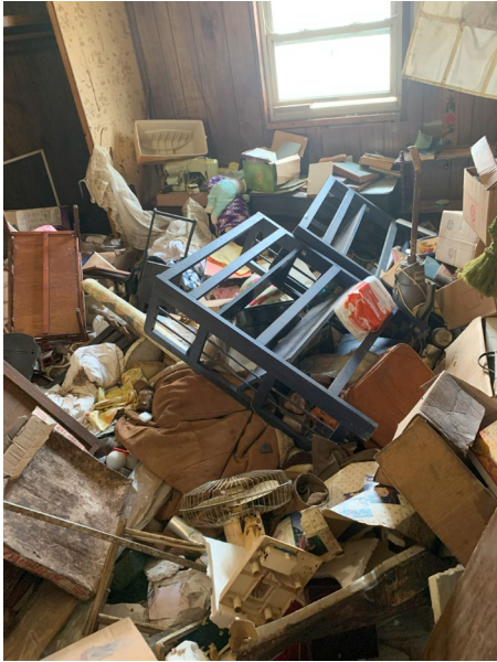
General Photo of Building Conditions
