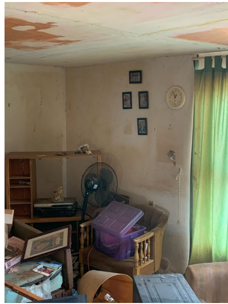
General Photo of Building Conditions
