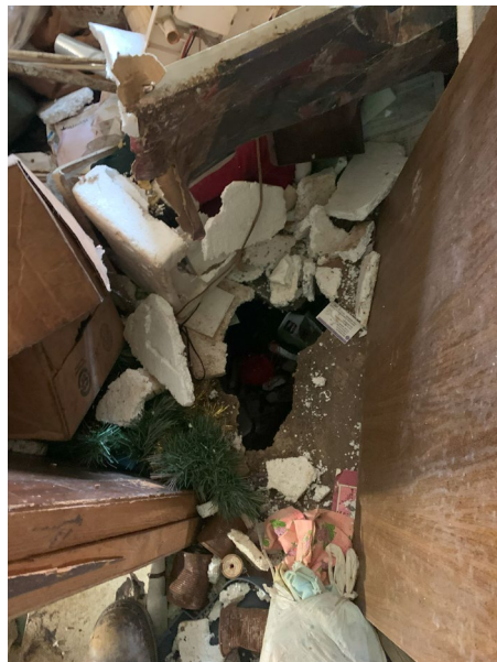
General Photo of Building Conditions
