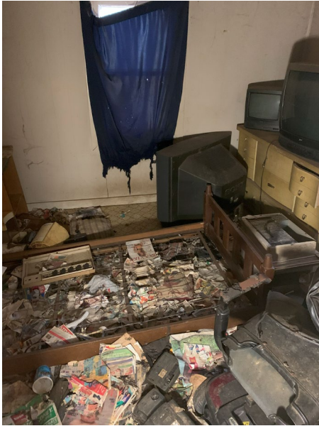
General Photo of Building Conditions
