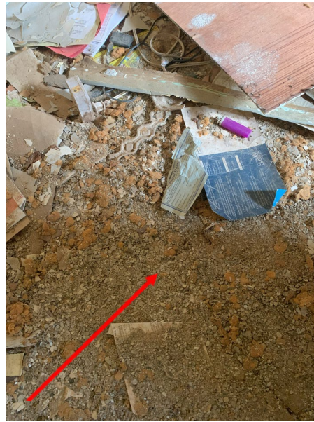
Assumed Asbestos-Containing Vermiculite
