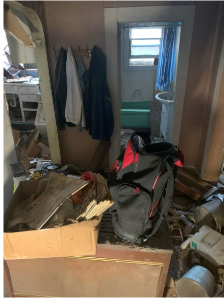
General Photo of Building Conditions
