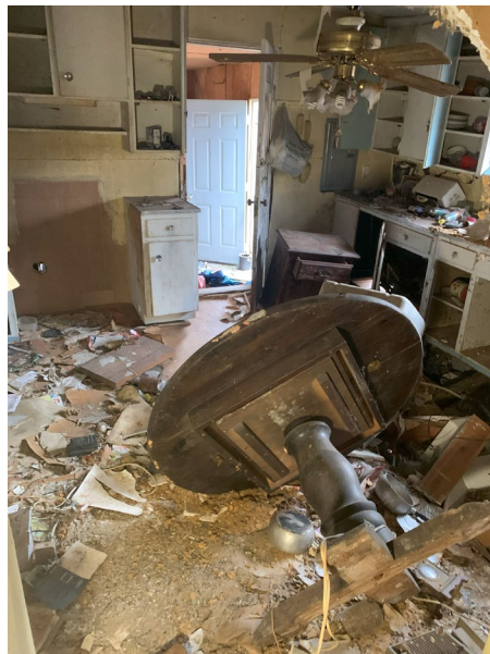
General Photo of Building Conditions
