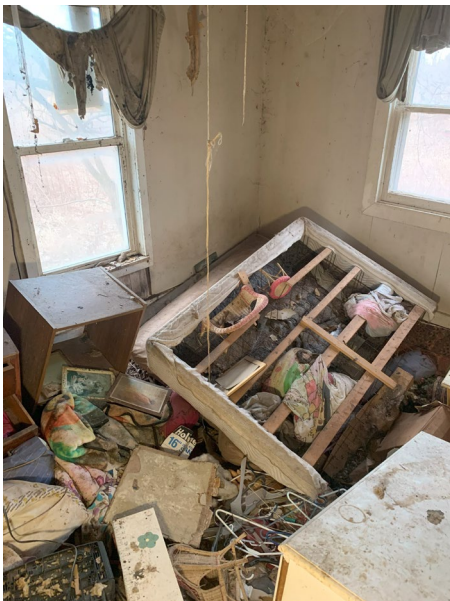
General Photo of Building Conditions
