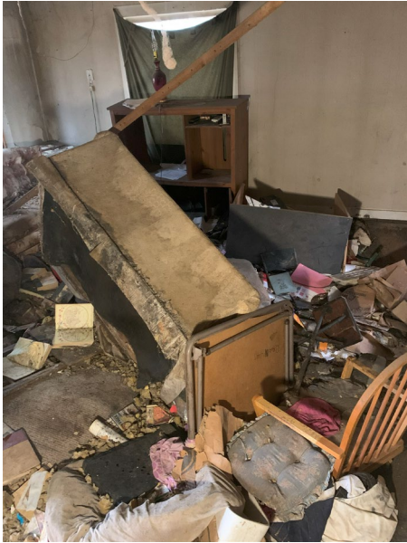
General Photo of Building Conditions
