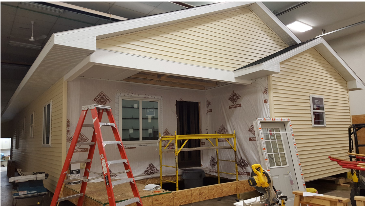
Mundy Charter Township - New Construction - $70,000
